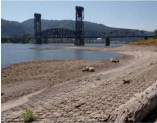
**Figure 2.** Exposed ACB and sand cap armoring at the McCormick & Baxter site.
