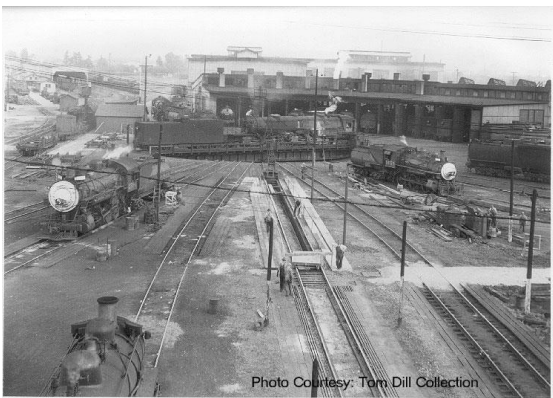
The historic Locomotive Maintenance Facility and Roundhouse.
