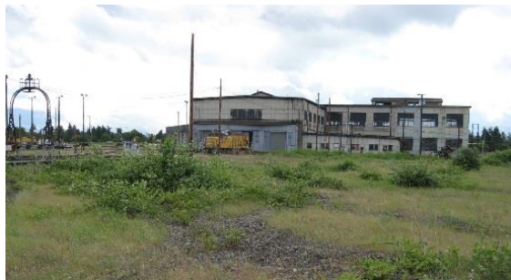
The Locomotive Maintenance Facility today
