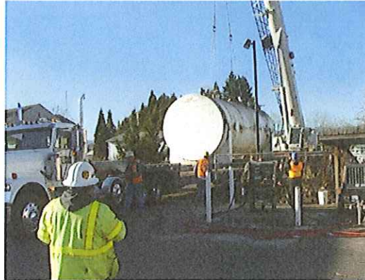
DEQ coordinates removal of gasoline and diesel above-ground fuel storage system.
