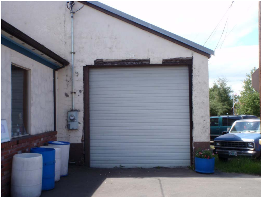
Photo 2: Roll up doors on the east side of the building
