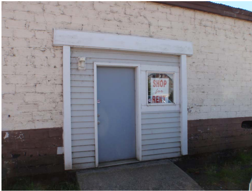
Photo 3: 2004 installed "man-door" on north side of the building
