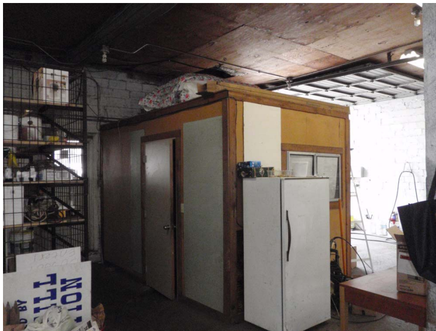
Photo 6: Showing interior modification
