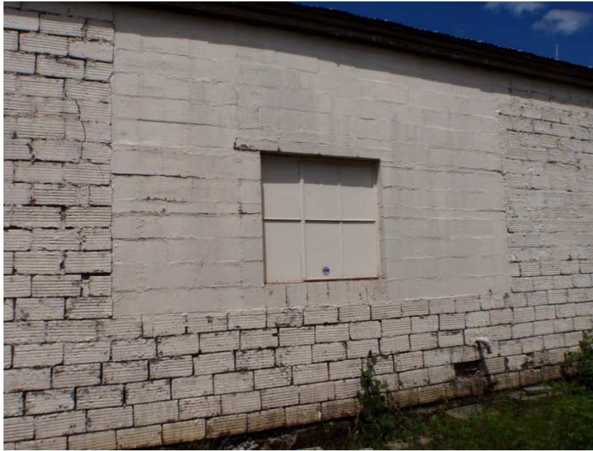
Photo 5: South side of building showing side window replacement
