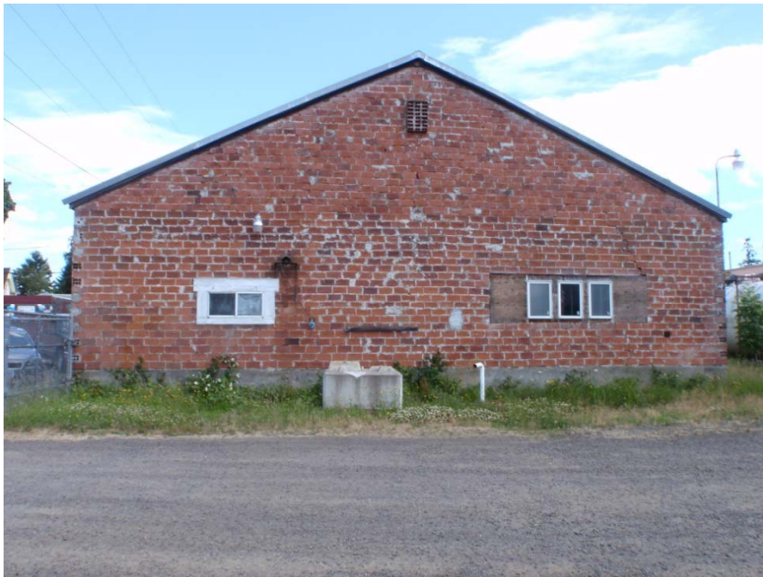
Photo 4: Rear window replacements, west side of the building
