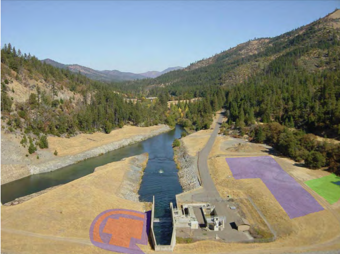
Figure 8. Photograph showing locations of project features and disturbance in relation to local vegetation (features are not to scale in this view). Purple represents disturbed areas which will be replanted (including the staging area); green represents the proposed vegetation mitigation area; and, orange represents the proposed powerhouse and access road.
