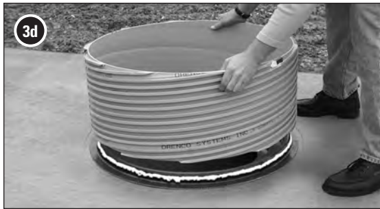
Carefully slide the riser onto the adapter.
