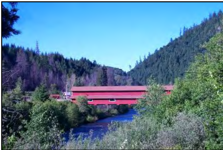
Covered Bridge Crossing the North Fork Middle Fork Willamette River in Westfir
