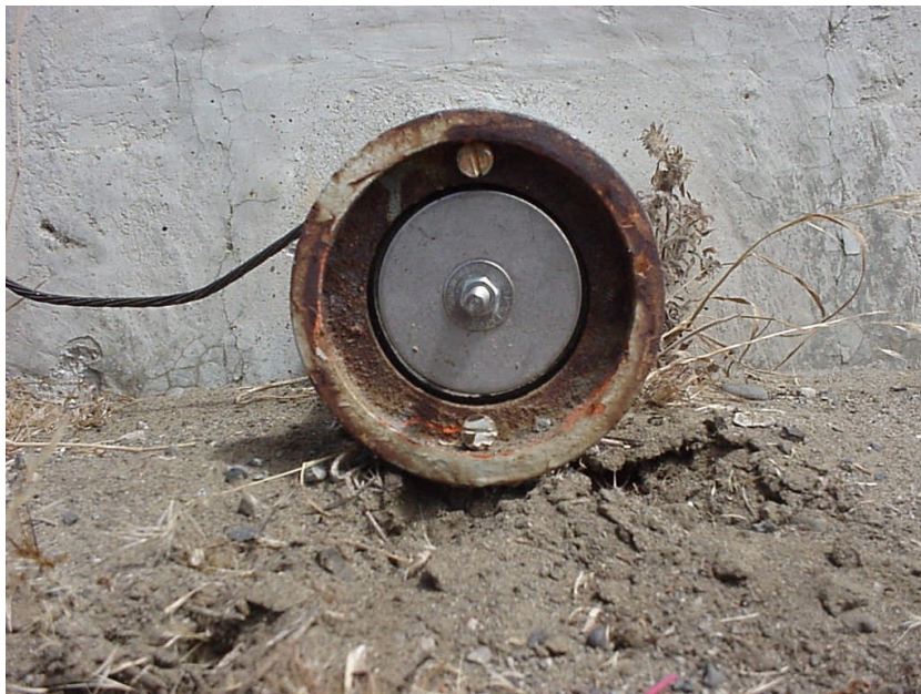
Floor Drain Plug Hex Nut Assembly
