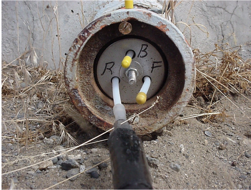
Floor Drain Monitoring Port Assembly
