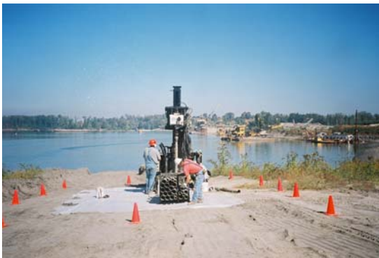
Installation of multi-level sampling well
