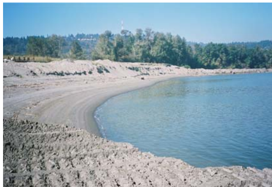
Southern shoreline where fill has recently been placed
