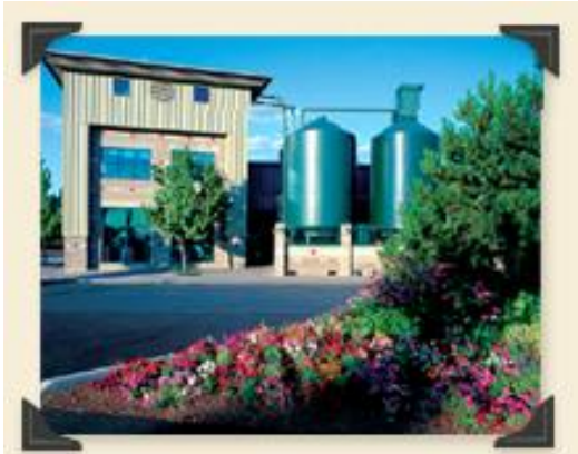
Deschutes Brewery Production Facility in Bend, OR
