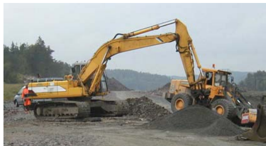
Many types of diesel engines can be retrofitted.
