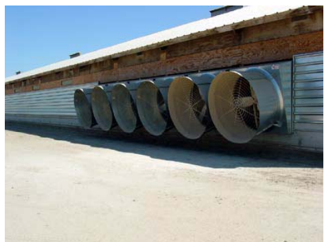
Totally enclosed, mechanically ventilated (Poultry Barn)
