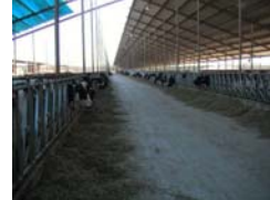
Partially Enclosed and Naturally Ventilated
